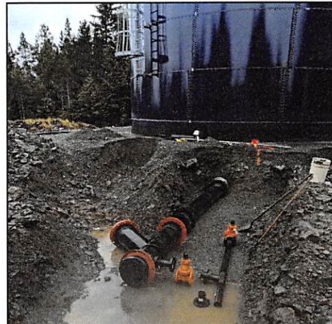
Reservoir Inlet / Outlet / Bypass / Swab Launch Piping
